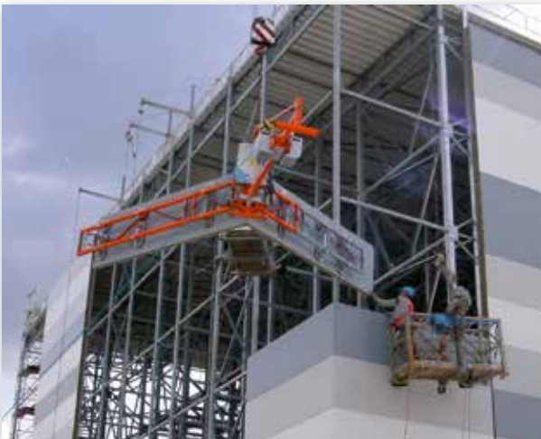
Special design of the OKTOPUS® Panel-Jack KT-B with counterweight system for the installation of corner elements
