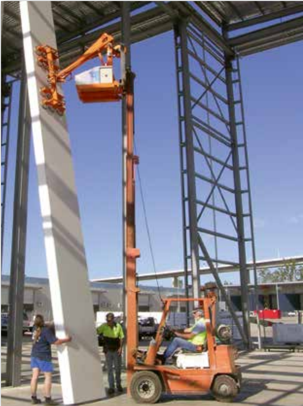
Installation of vertical wall panels with the OKTOPUS® PANEL-Jack GI-B400
