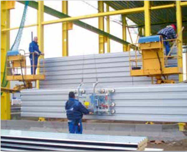
OKTOPUS® Panel-Jack KT-B with oval suction cups for the installation of trapezoidal elements
