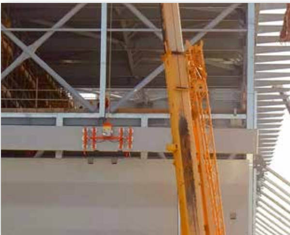
Installation of horizontal wall elements with the OKTOPUS® Panel-Jack KS-B
